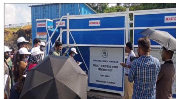
Expert interacting with the trainees at the Mobile Faecal Sewage Treatment Plant, Port Blair
